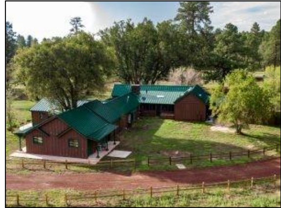
Figure 2: View of the historic Hut Ranch
